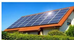
Solar panel installations
