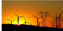
Upgrading the power grid
